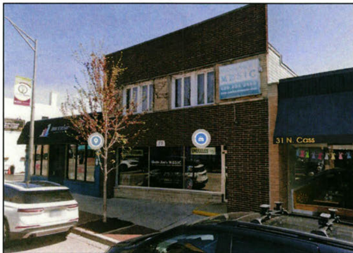
33 North Cass Avenue (street view - Source: Google - prior to destruction)
