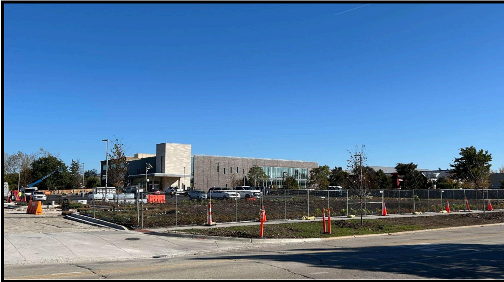
AOC construction progress (view of northwest corner) - October 2025
