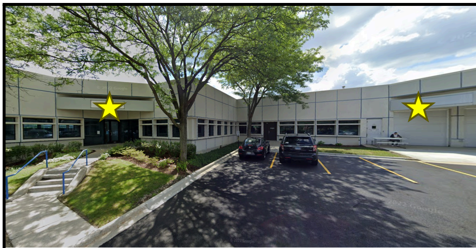
View of the Unit from the North Side - 600 Oakmont Lane, Suite 600 (source: Google) (stars mark access points to the subject unit)
