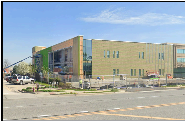
Street View from Ogden Avenue (under construction) - 639 Blackhawk Drive (source: Google)
