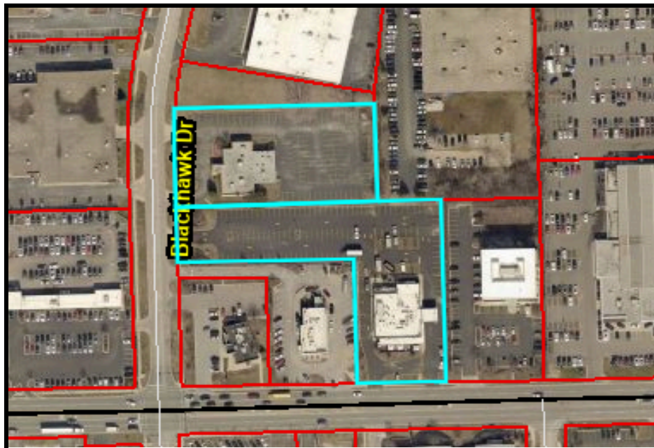
Aerial Map - 639 Blackhawk Drive and 330 East Ogden Avenue (prior to redevelopment) (source: DuPage County Parcel Viewer)
