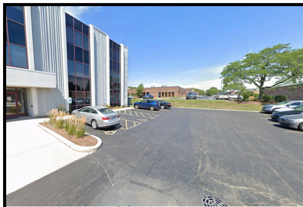
View of the Proposed Generator Location - 801 North Cass Avenue (source: Google)
