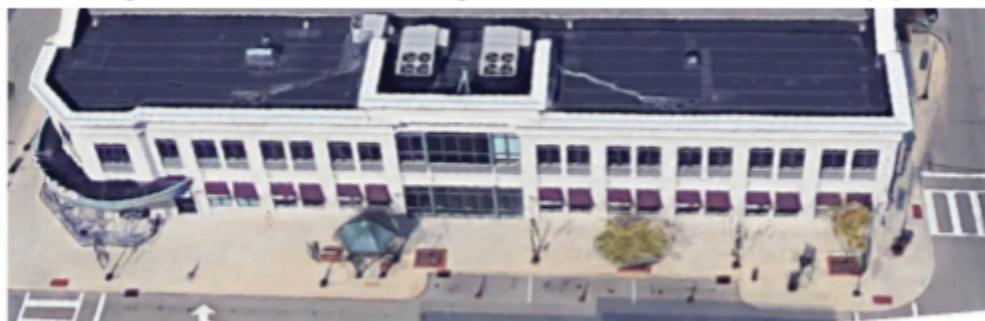
Rooftop Utilities Screened from the Public Way by a Parapet
