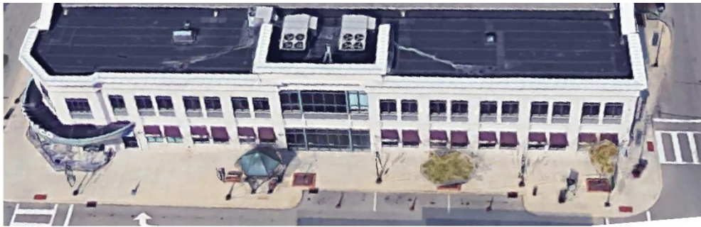
Rooftop Utilities Screened from the Public Way by a Parapet
