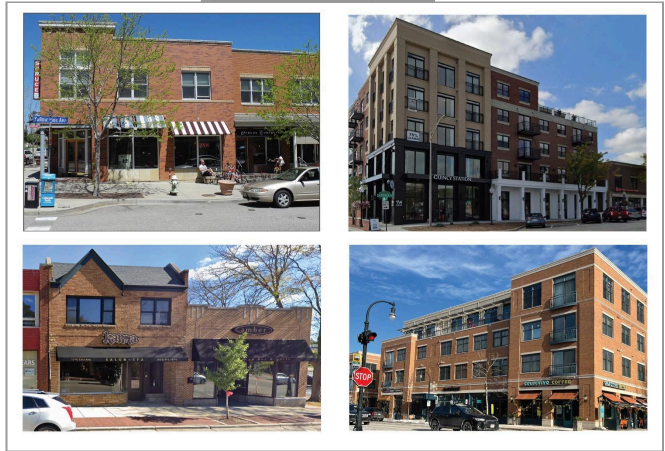
Figure IV-1: Storefront Building Examples
