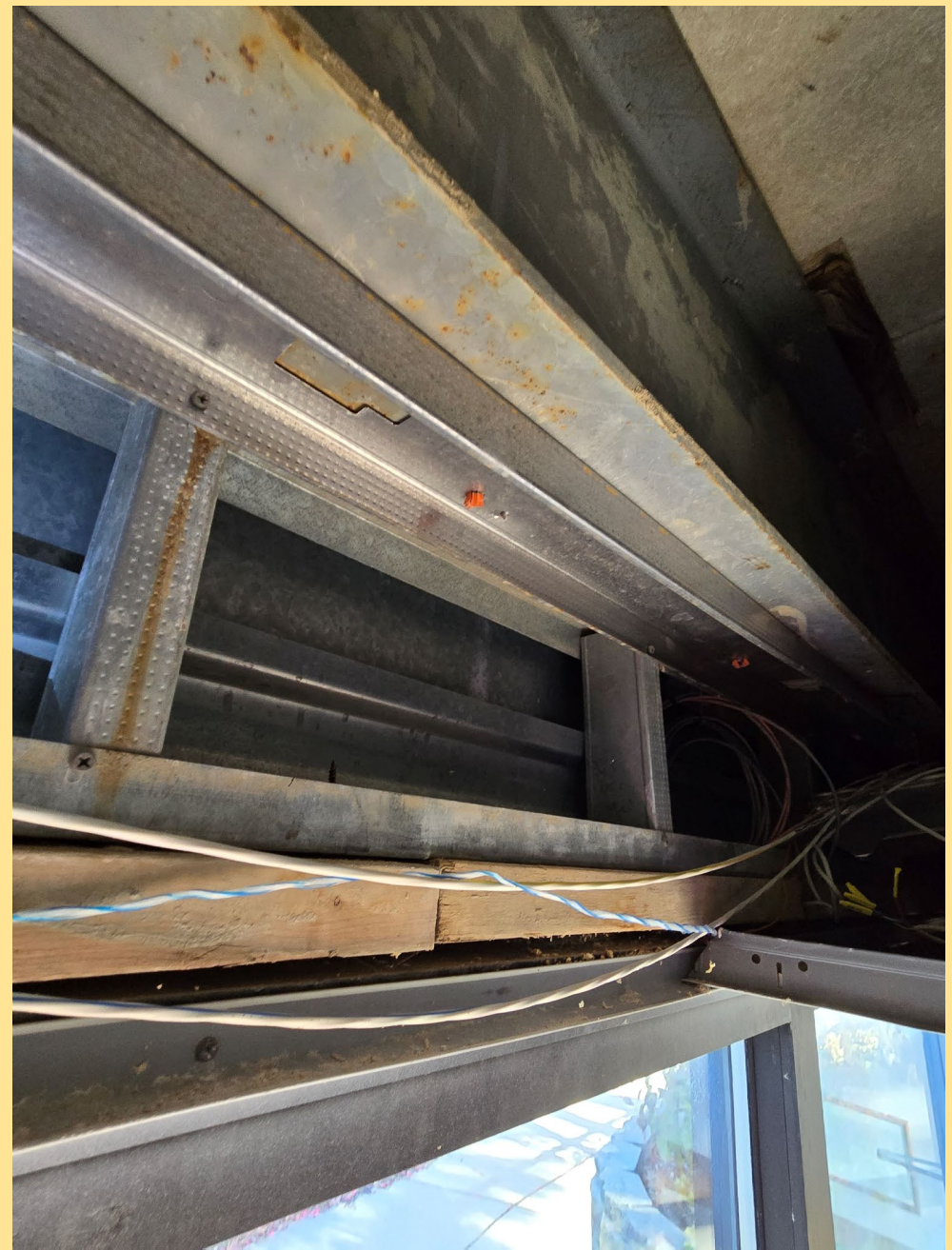
SOUTH ELEVATION- VISIBLE DAYLIGHT COMING THRU FACADE
