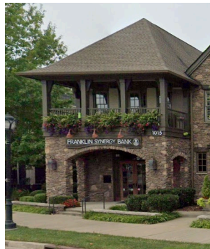
Balcony as an extension of the building, sharing roof structure.
