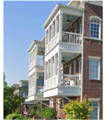
Stacked balconies with visible support structures.
