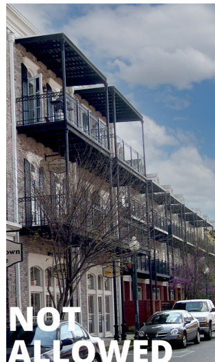
NOT ALLOWED Balconies: Covers More than Allowed Facade Area
